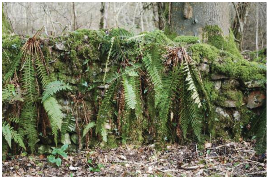
FIGURE 4 Detail of the north wall
