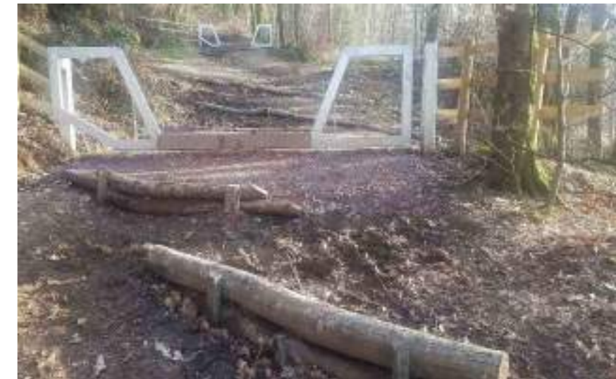
Example of the woodland tracks where heavy erosion and 4x4 use was contributing to sediment run off and overland flow. Closure of path to vehicles under a DCC issued Flood Prevention Order and installation of horse-friendly barriers & natural 'grips' to send water into the woodland floor.
