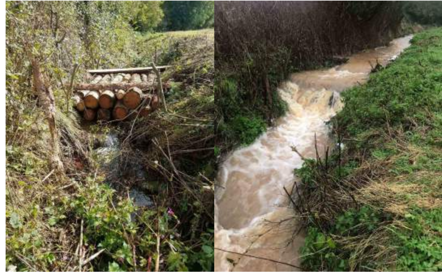
An example of a longitudinal leaky dam in the watercourse. Dam designed to retain water in channel. LEFT: on completion (Oct 19) RIGHT: during Storm Dennis (Feb 20)
