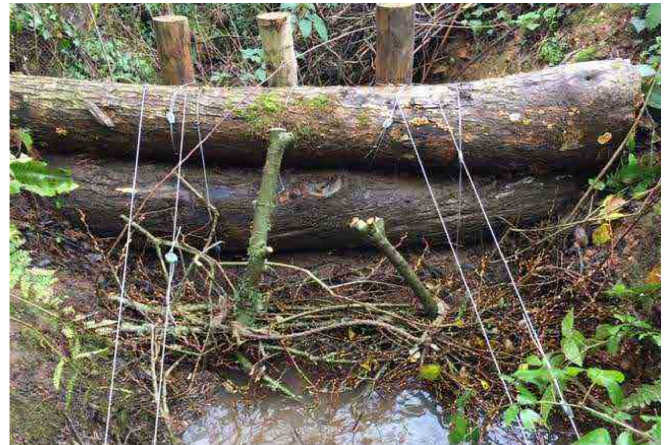
Example of cross-channel dam. Image: © Devon Wildlife Trust
